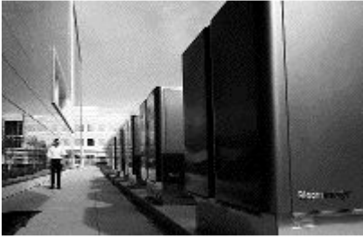
A bank of 'Bloom Boxes' powers eBay headquarters in San Jose, Calif.
