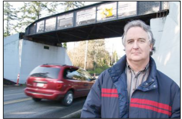
Drivers should be prepared for delays along Island Highway this year as View Royal launches a major overhaul of the commuter artery, says View Royal engineer Emmet McCusker. Traffic will be limited to one lane between 6 a.m. to 3 p.m. starting this week.
